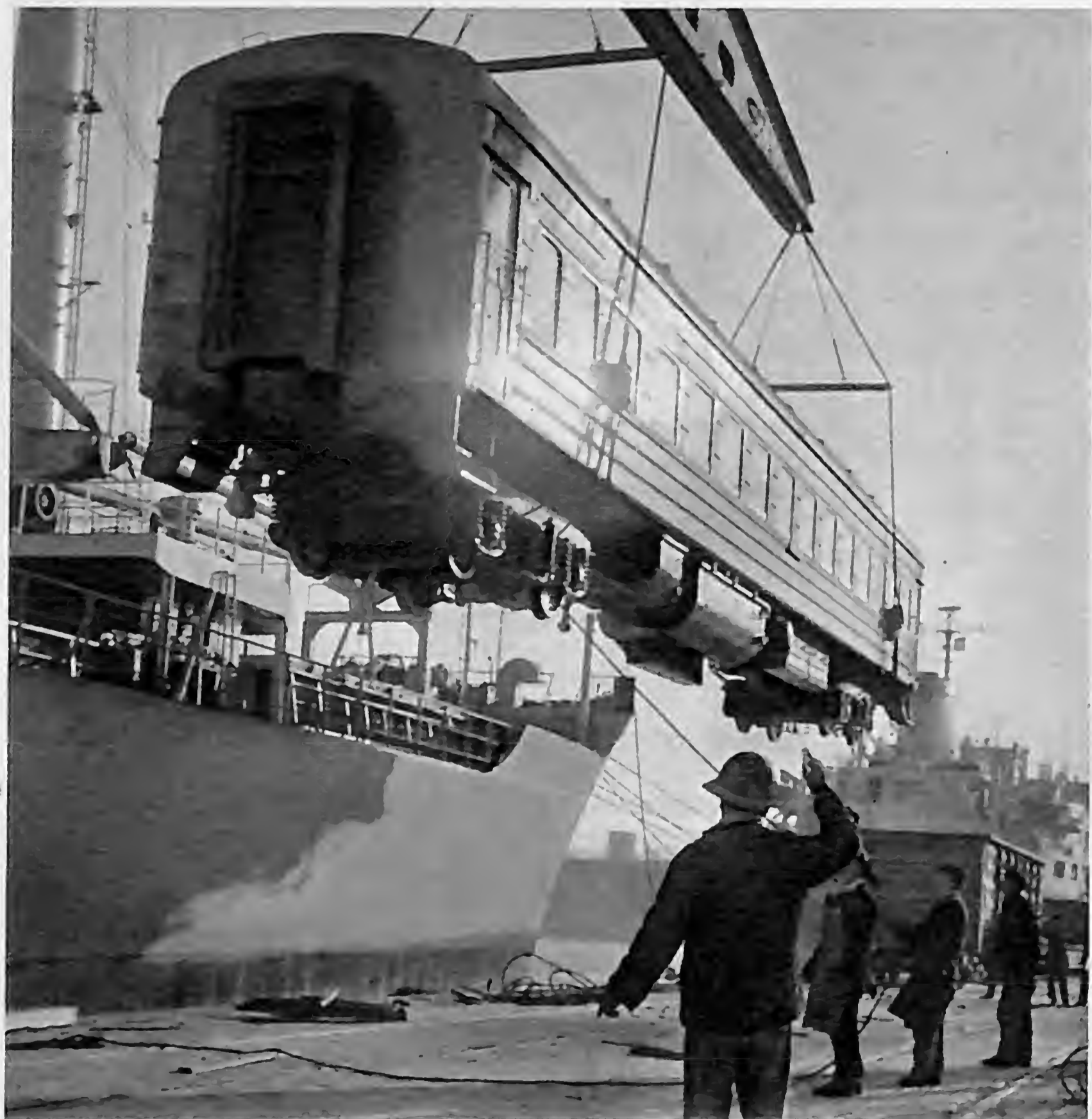
Loading a railway coach on board ship.
